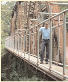
Luis Diego Chacón, head of EARTH's transportation group, was instrumental in the construction of the walkway. Since this photo was taken in December, community members completed the walkway, finishing the installation of chain-link fencing on both sides and painting the structure.
